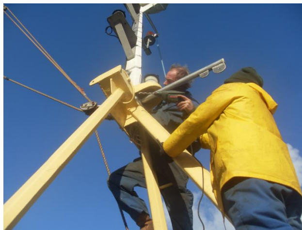
Figure 1: The fabricated fitting being bolted to the tripod mast
