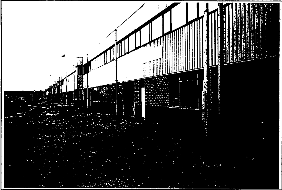
Figure 3 - Ijmuiden New Processing Units - external view of rear
