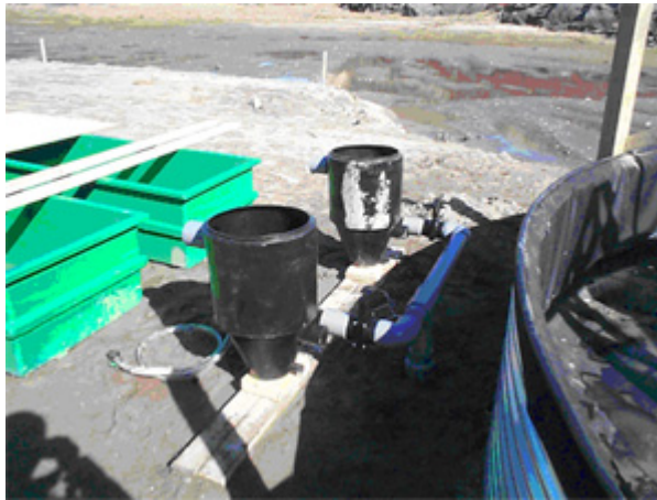
Image 2 Installation of Swirl Separators
