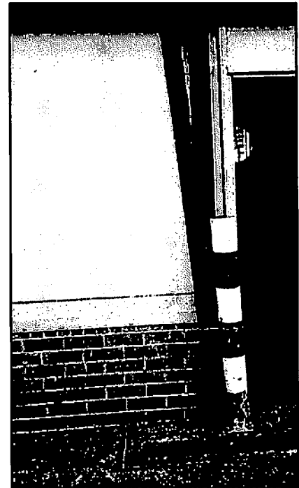
Figure No. 7 - Damaged downpipe outside the fish market
