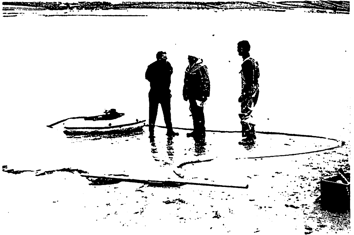
3. Water jet and pump used for inserting buxhot poles.
