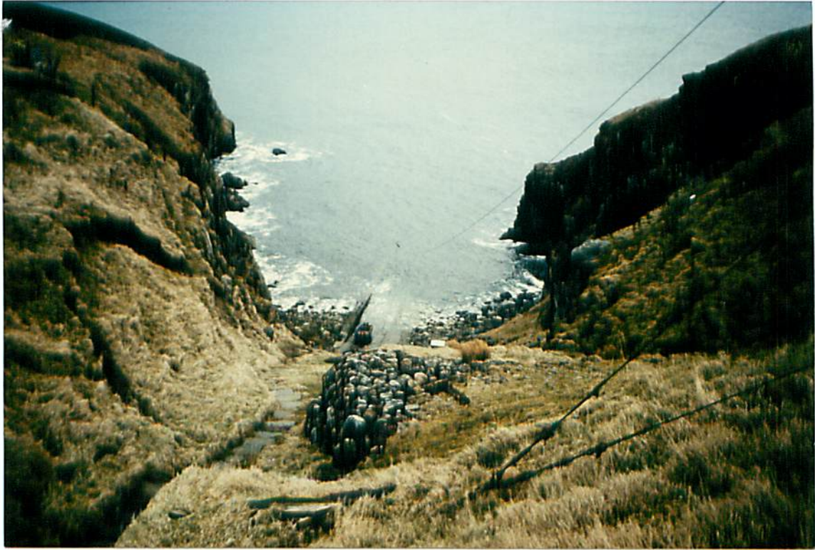
Photograph 13 - Port Grant Boat Hoist
