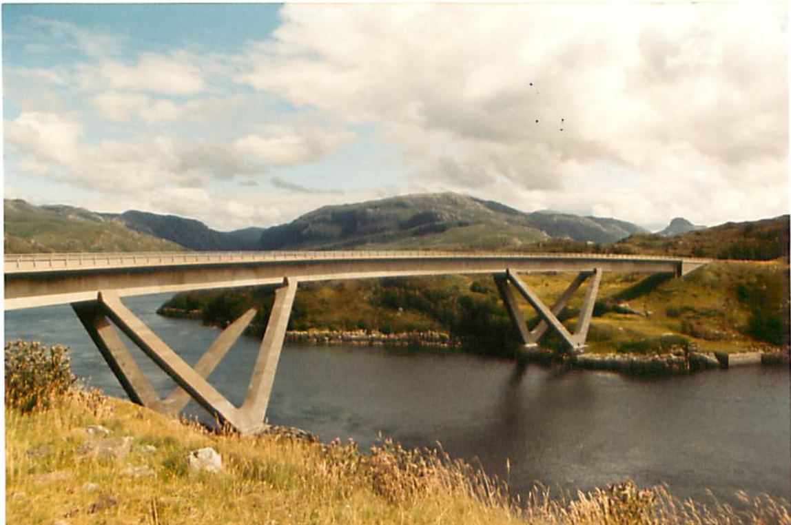
Photograph 10 - A894 Kylesku Bridge
