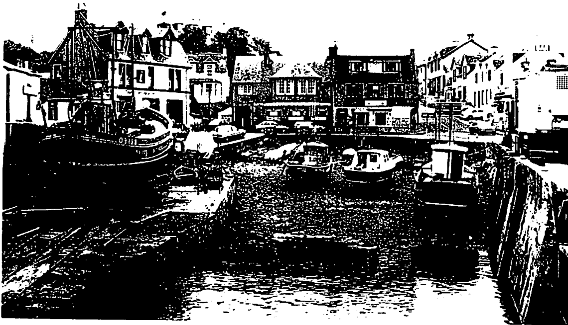
Photograph 6 - Mallaig - Boatbuilding Slipway
