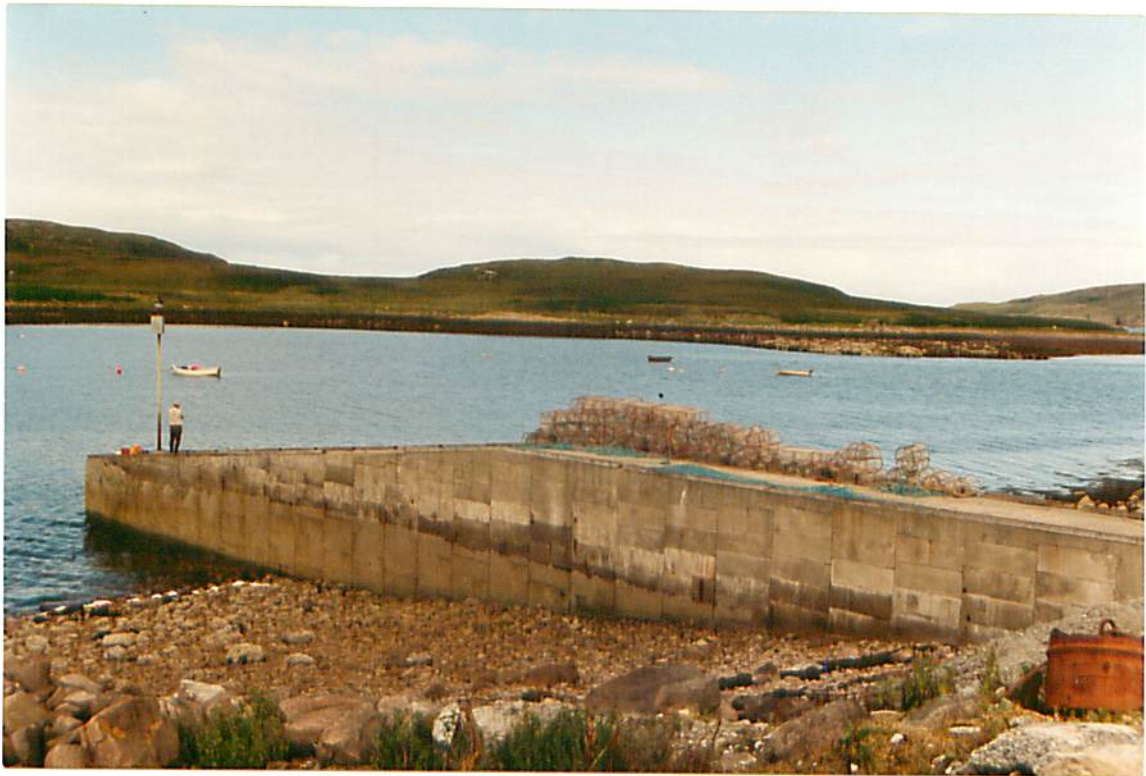
Photograph 16 - Old Dornie - New Pier
