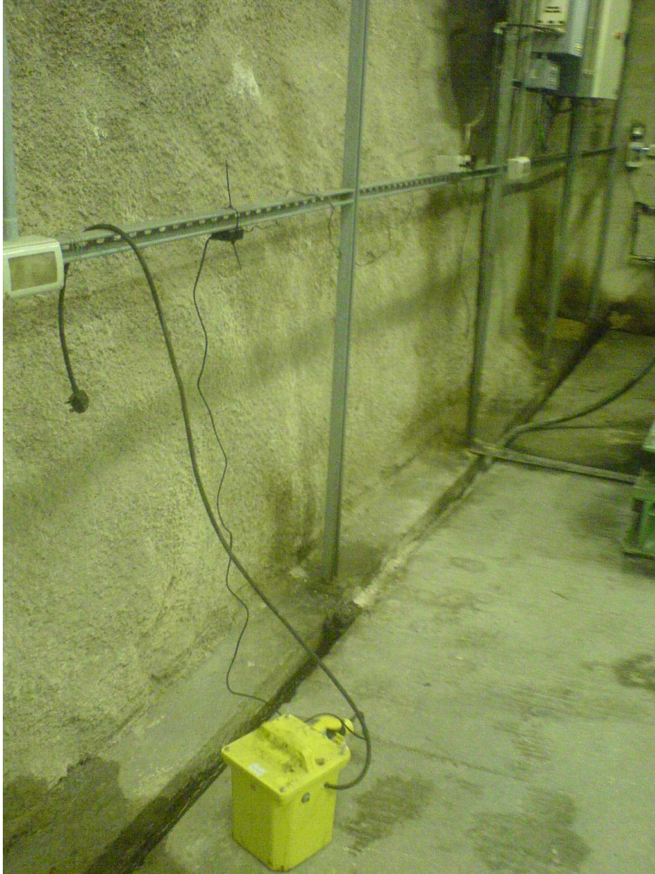
Figure 04: General arrangements for the FuelVantage Digital Fuel Treatment system (N.B. Yellow Transformer disconnected from supply for 'before' DayTrawl test)
