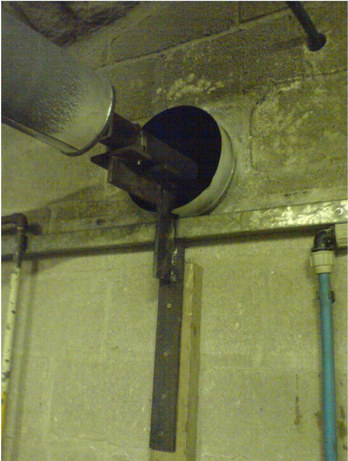
Figure 03: Exhaust extraction arrangements after comparative testing with Vaughan Industries FuelVantage electromagnetic system but before developmental testing for Vortex Performance Exhausts Ltd
