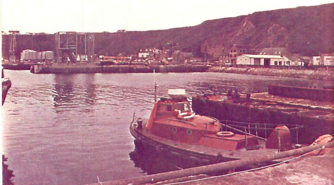
Photo 5 - Ferry basin with new ice store in background.
