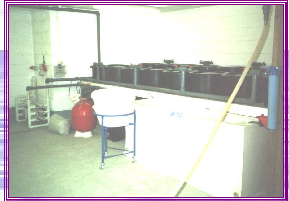
Typical 70 L conical vessels, suitable for turbot egg incubation, with a simple recirculation system, sand filters and 1 micron cartridge filter
