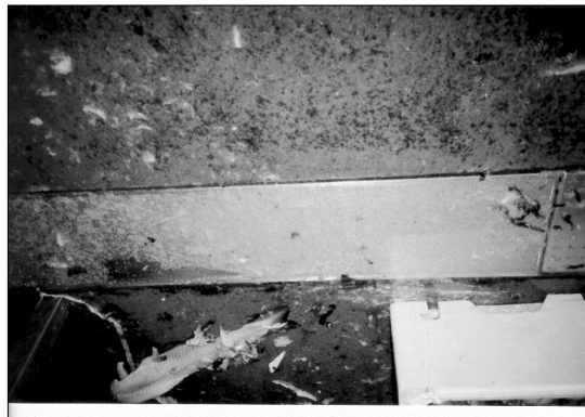
Figure 25 - 0.5mm Aperture Wedge Wire Drain Cover (16% open area)
