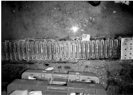
Figure 24 - Original Slotted Drain Cover (40% open area)
