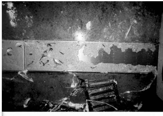
Figure 26 - 1mm Aperture Wedge Wire Drain Cover (27% open area)
