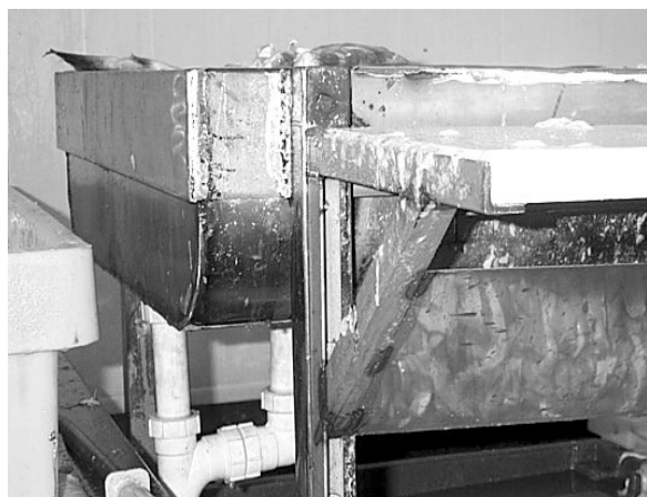
Figure 7a - High Capacity Overflow Arrangement
