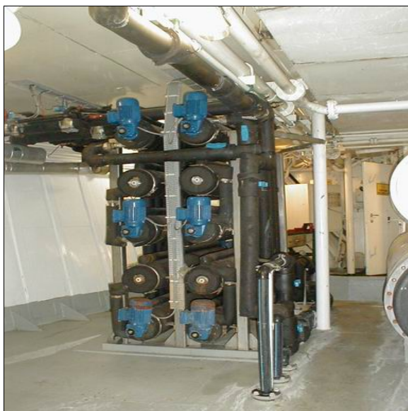
Figure 2 - Installation of 10 binary ice making cylinders on a large pelagic vessel
