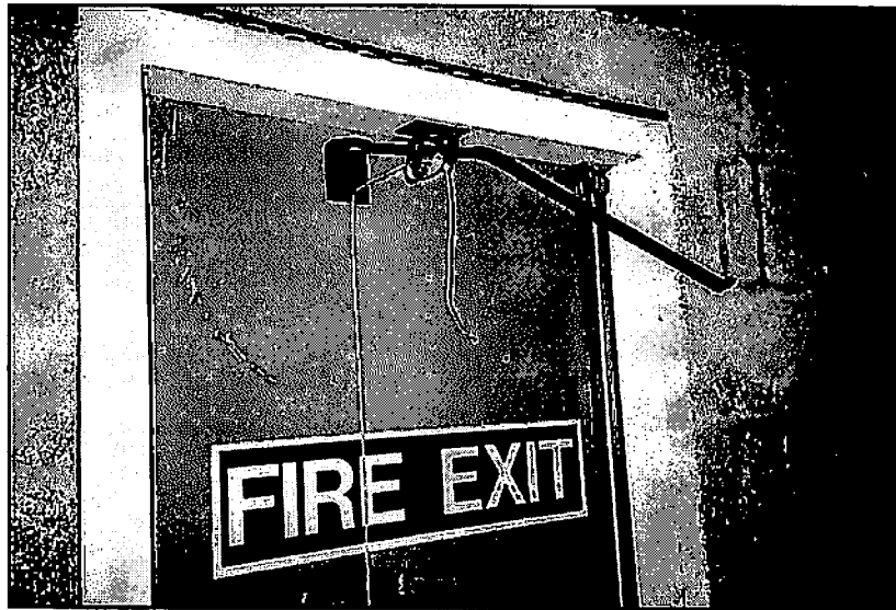
Figure 10 - Damage to the doorway stays
