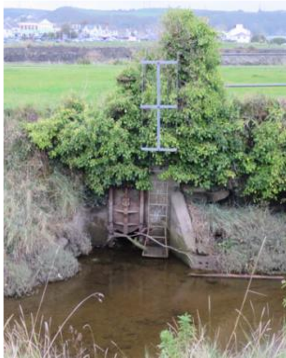
Plate 25: Combined sewage outfall (CSO) at Burry Port, Burry Inlet
