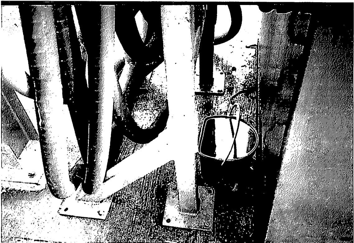
Figure 19 – A bucket is used to catch fuel from a leaking pipe
